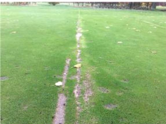
Figure 17: Some work is still required to regain grass cover and surface levels over the drain lines. This will be easier in some areas than others but the greens should now be appropriately rested to allow for recovery.
