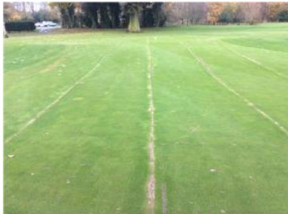
Figure 16: Drainage installation to the 9<sup>th</sup>, 11<sup>th</sup>, 13<sup>th</sup> and 15<sup>th</sup> greens has been a resounding success and has already notably improved surface drainage and firmness. Organic matter reduction will further improve drainage performance.
